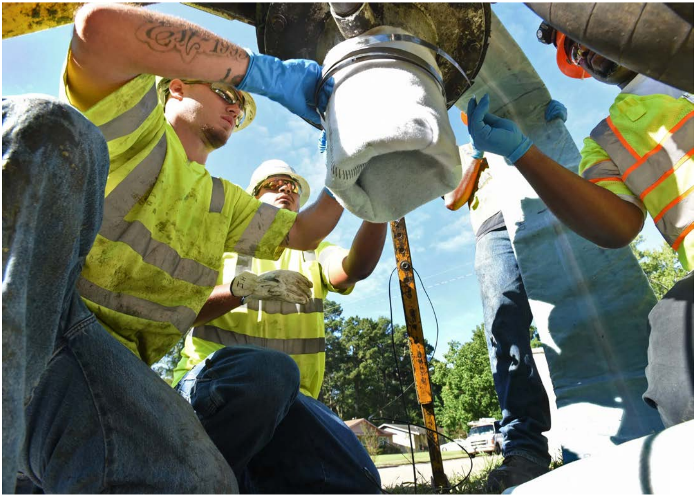
Members of an Insituform CIPP installation crew prepare to feed a resin liner into an old sewer pipe in Shreveport, Louisiana.
