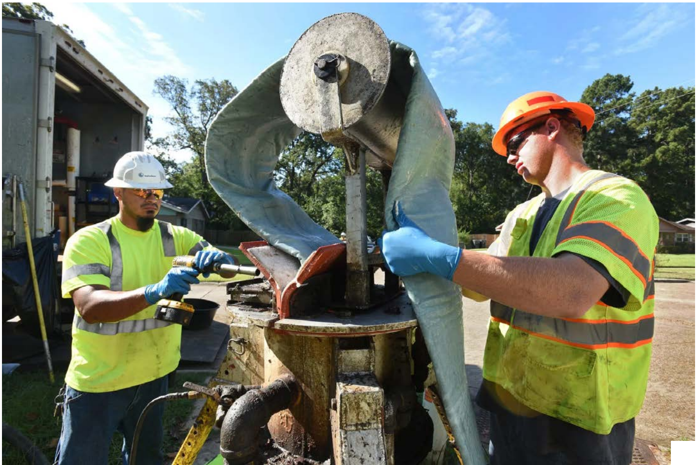
Members of an Insituform CIPP installation crew feed resin liner into an old sewer pipe in south Shreveport, Louisiana, in 2017.
